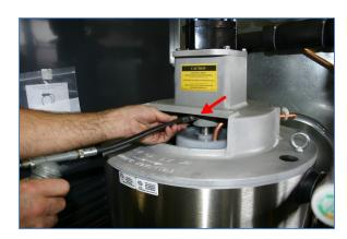
Typically, only one squirt of the grease gun is required or until you feel resistance on the pump.
