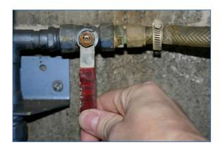
4. Close water supply at shut-off valve.
